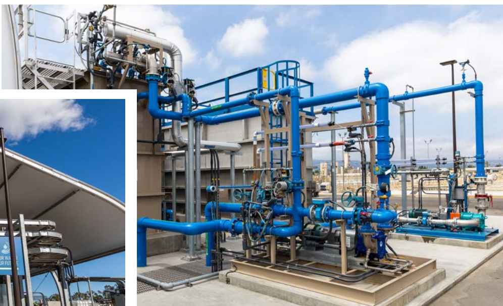
Membrane bioreactors at the Regional Recycled Water Advanced Purification Center
